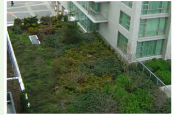
Absorbent landscapes like green roofs
