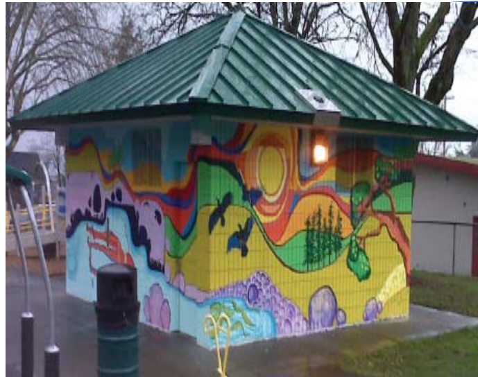
The washroom pavilion in Deverill Square Park was painted by community members.
