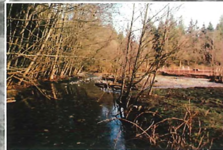
The diverted channel above lacks riparian vegetation and is adjacent to livestock fields. Fish habitat may be damaged by bank erosion and water contamination.
