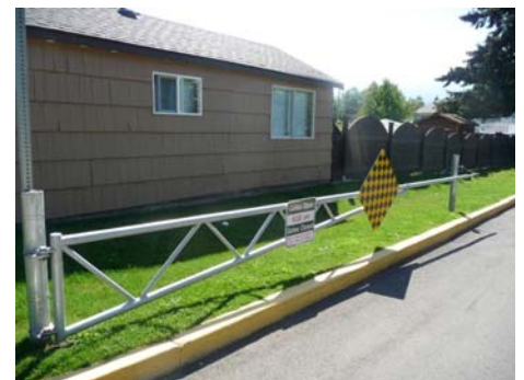
New gate to control access outside of park hours.
