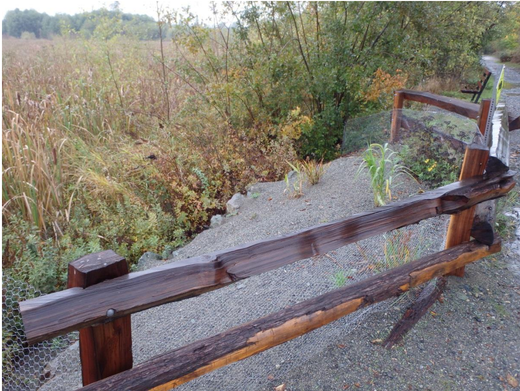
Turtle nesting area on dike at east property boundary
