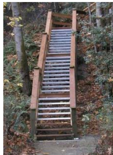
Stairs near Bradley Street. Treads are metal and have great traction.
