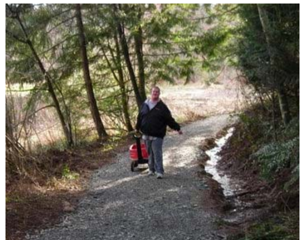
Drainage swales are evident on the uphill side of the trail in Linley Valley (Cottle Lake) Park.
