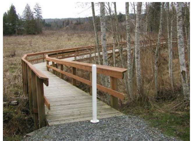
Raised boardwalk at Richard's Marsh (above and left) ties into the local trail system and leads trail users on a direct path across the marsh. The marsh was previously a barrier and the boardwalk now provides access to the local school and recreation amenities.
