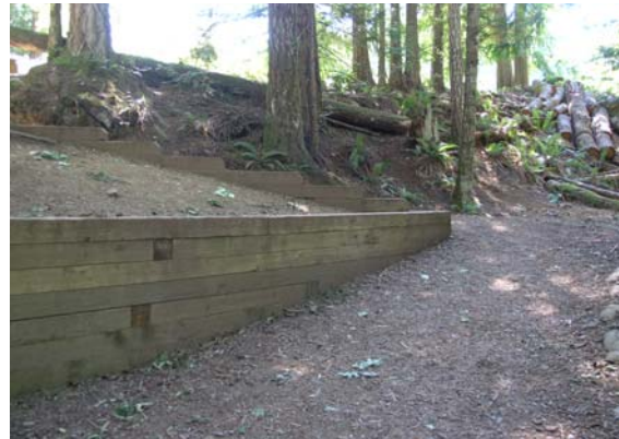
Example of a retaining wall along the Westwood Lake Trail.
