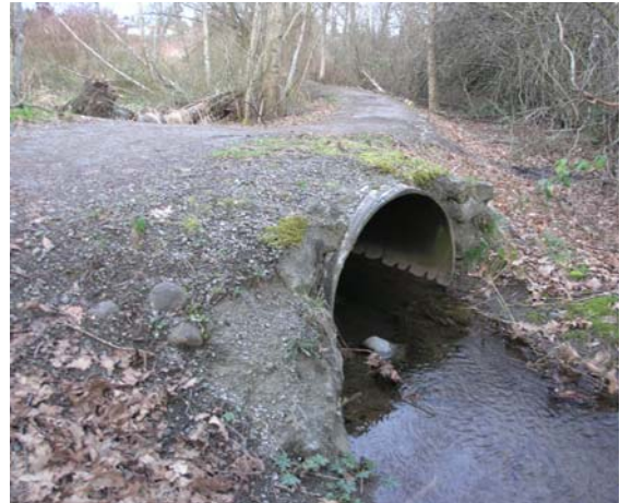
Culvert and headwall at Buttertubs Marsh.
