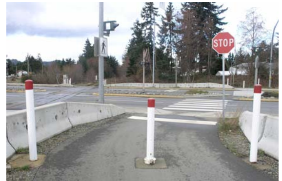
Signalized trail crossing with a raised median island to allow safe crossing of Mostar Road for E&N Trail users.
