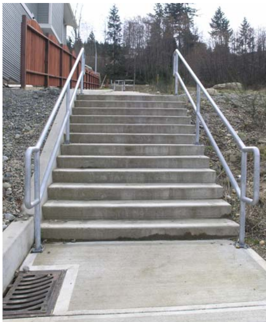
Concrete stairs (with railings, drainage, and vehicle barriers) in the Gulfview neighbourhood.
