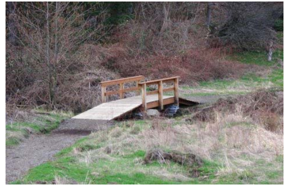
Trails in Nanaimo are kept at a 3% grade as much as possible with good drainage to keep trail users dry and trails in good structural shape.
