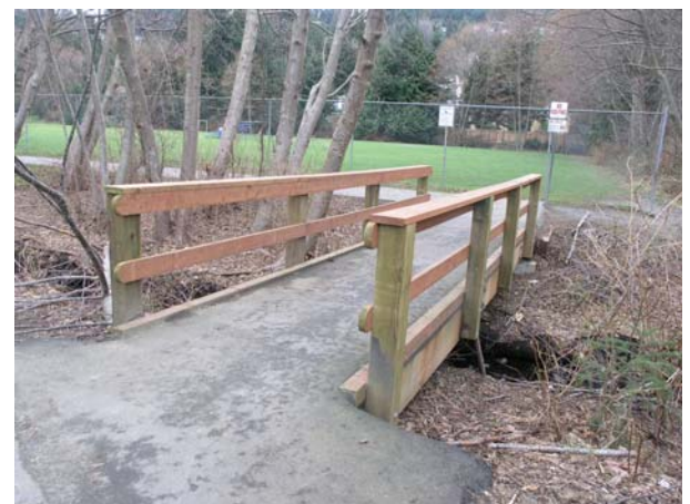
Paved bridge along Walley Creek provides continuous multi-use surfacing material.
