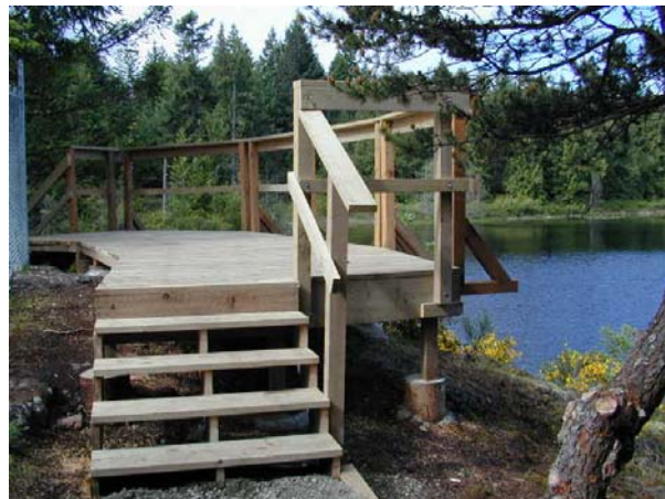
Wooden viewing platform and bridge along the Lost Lake Trail.
