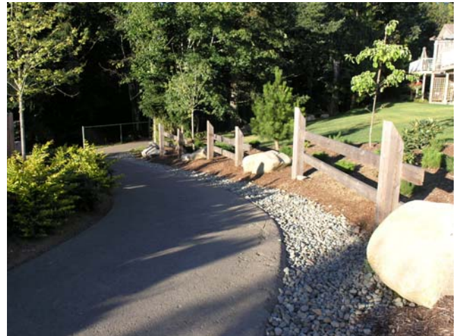
Low wood rail fencing along the Rutherford Ravine Trail delineates public and private space.
