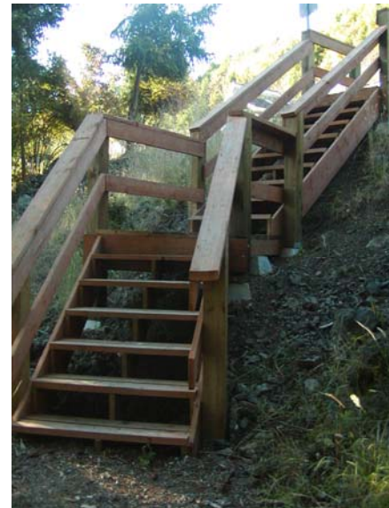
Stairs at Fillinger Waterfront Park. Staircases are appropriate for high use trails.
