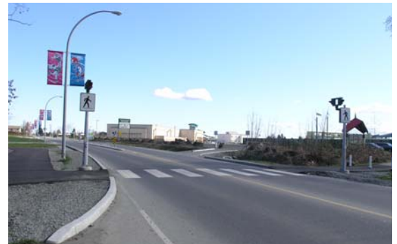
Signalized trail crossing at Third Street provides a safe road crossing for trail users.
