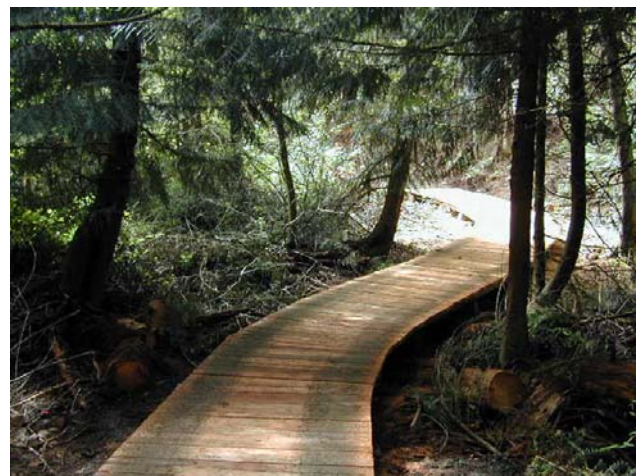
Boardwalks like this one at East Lake Park elevate trails to lead trail users over wet locations.
