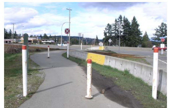
At-grade crossing of the E&N Trail near Waddington Road is well marked with 3 sets of 3 post and sleeves.
