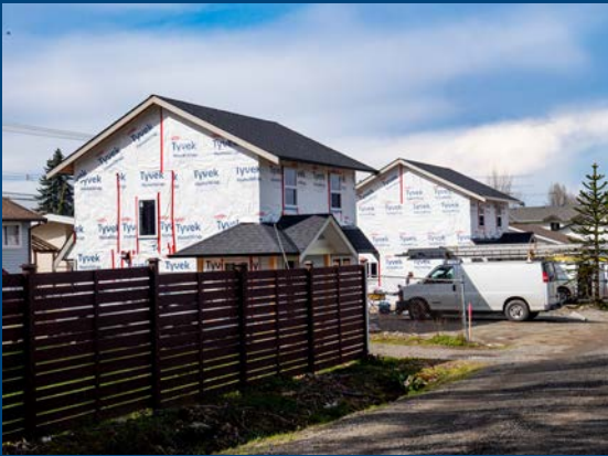
New carriage home construction
