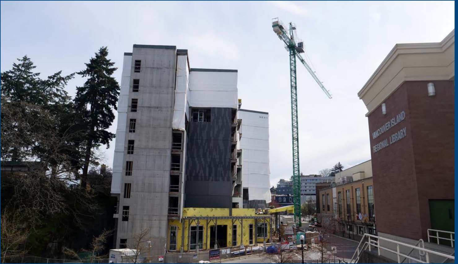
Construction of the new hotel on Gordon Street
