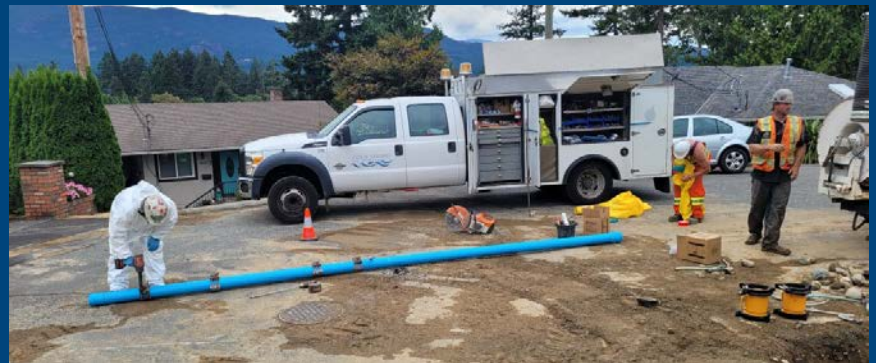
Water main repair on Bates Road
