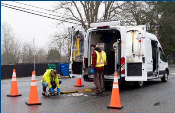
New sewer truck to assess conditions of sewer mains
