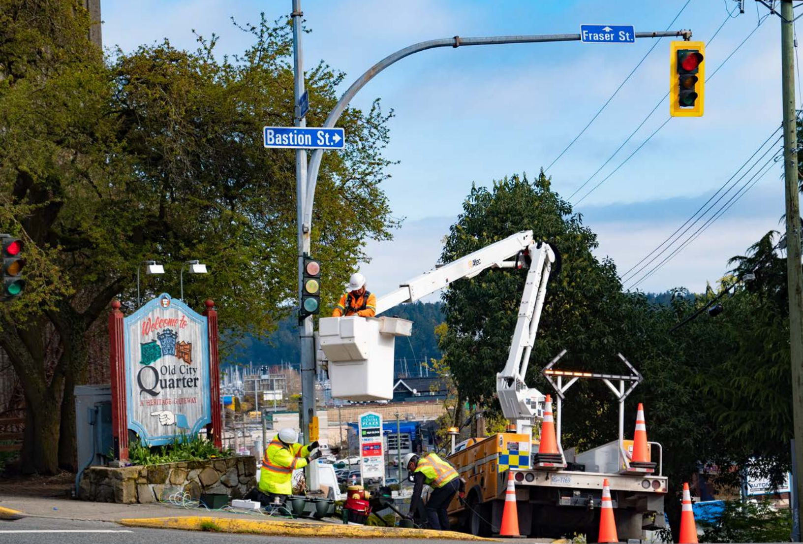
Crews working at the entrance to the Old City Quarter
