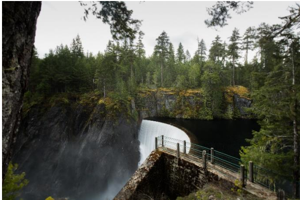
Raw water collected and stored in South Fork Dam
