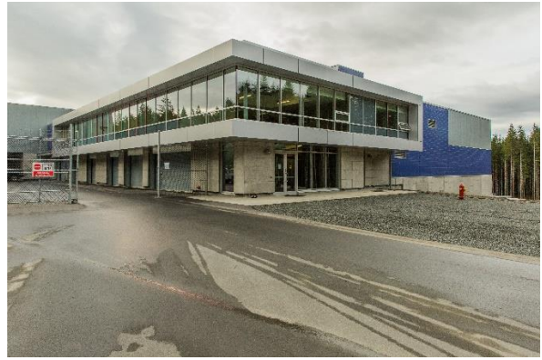
Raw water flows (by gravity) to South Fork Water Treatment Plant
