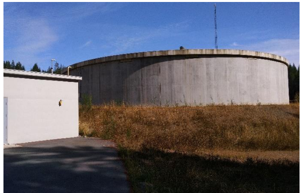
Treated potable water clearwell (storage tank)
