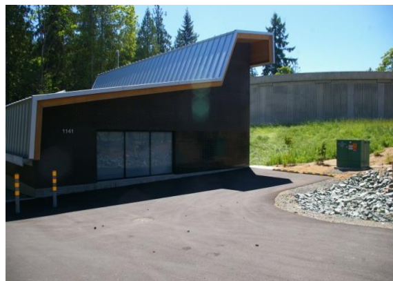
The Energy Recovery Facility and the Reservoir #1 drinking water storage tank (in the background)
