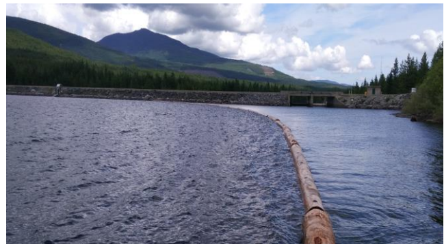
Jump Creek dam and log boom
