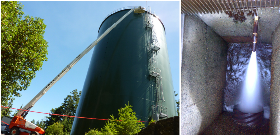
Figure 2-10: Photos of Duke Point Reservoir and Blow-Off
