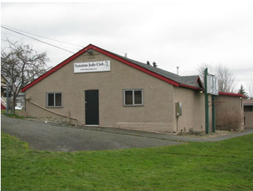
Name: Connaught Barracks Stable Location: 850 Wentworth Street Date: Circa 1915
