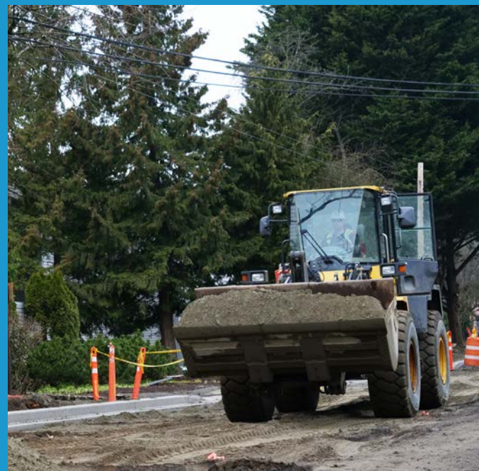
Metrol Drive Complete Street construction
