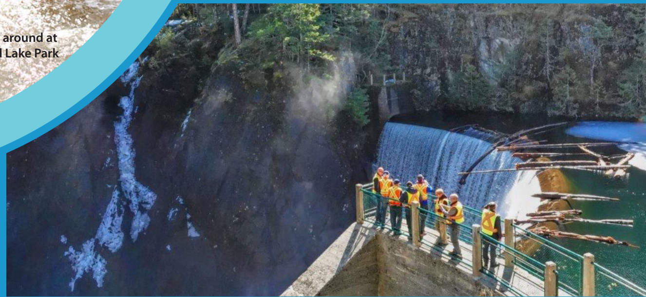
South Forks Dam
