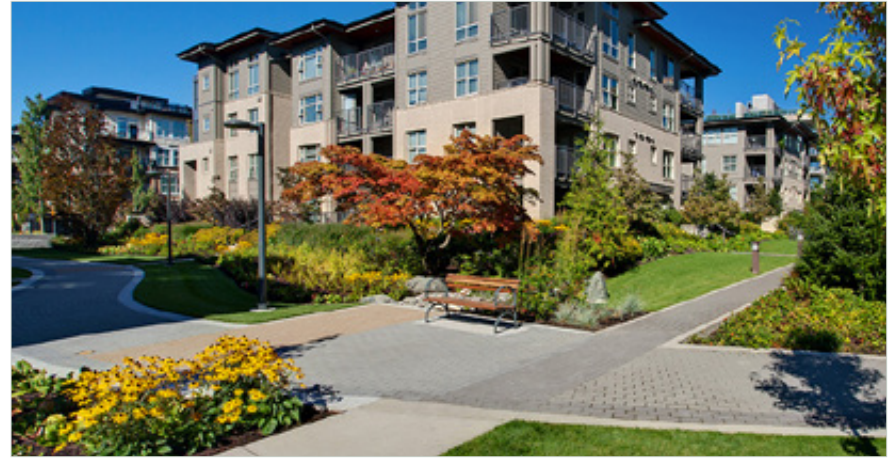
A greenway connection intersects with a sidewalk
