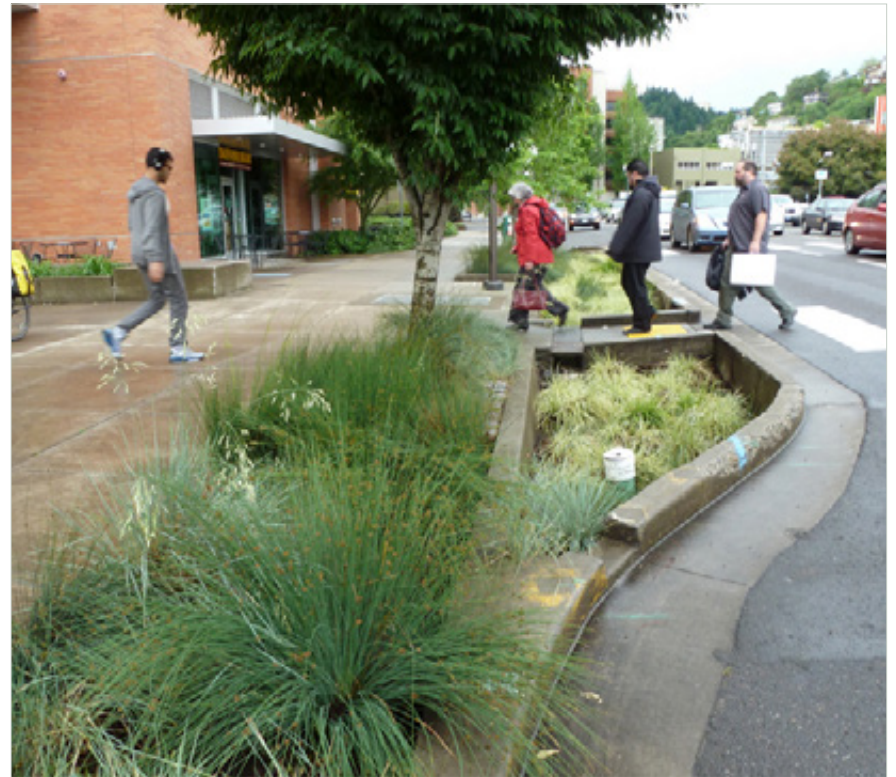
Curb extension with rain garden at crosswalk on village main street
