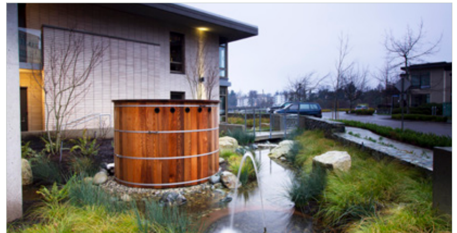
Utilizing greywater recapture for site-wide irrigation and a design feature
