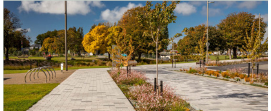
An example of permeable surfacing and soft landscaping area at the entry to a public park
