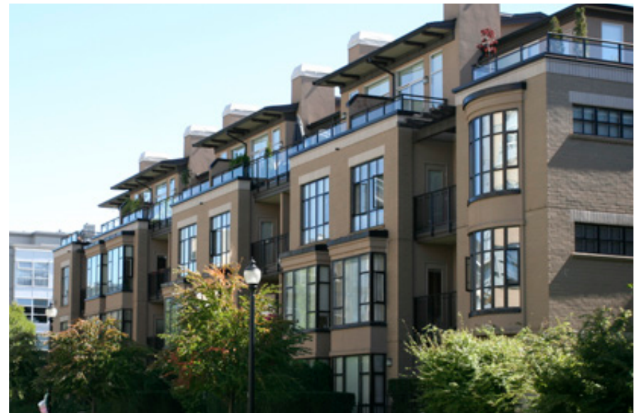
A building with a significant upper storey setback utilized as private balcony spaces
