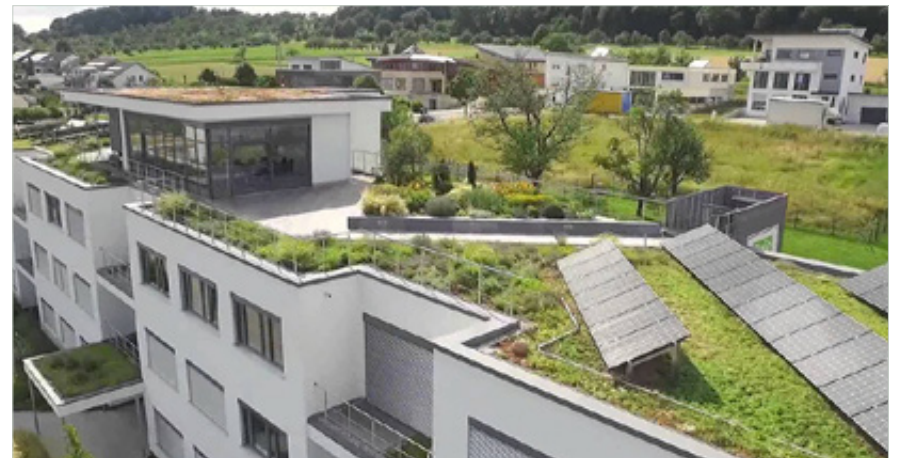
A residential building with accessible green roof and PV system
