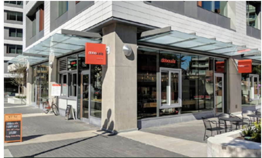
A RETAIL/COMMERCIAL BUILDING WITH ACTIVE STREET FRONTAGE
