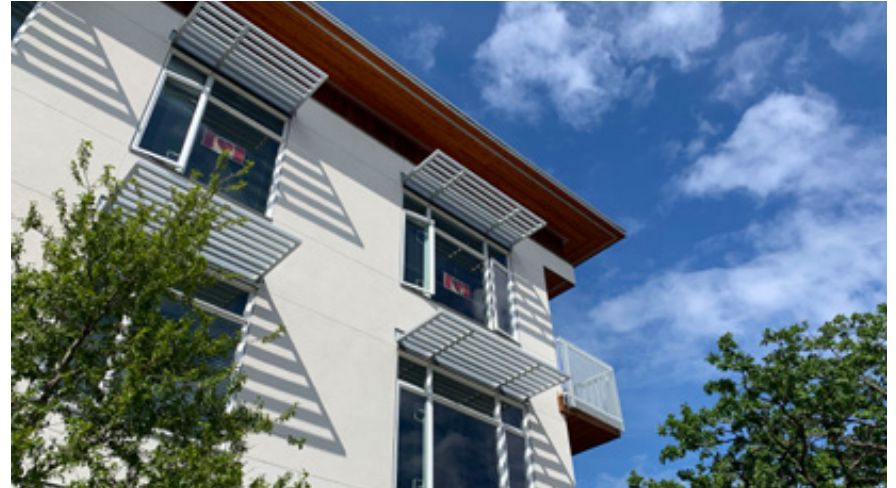
Exterior shading devices can be integrated into a building's southern elevation to block unwanted solar gains and keep indoor temperatures comfortable in warmer months.
