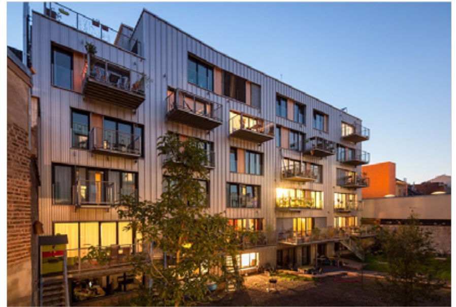
A high performance (Passive House, Step 5 equivalent) residential building with thermally broken windows and a low window-to-wall ratio
