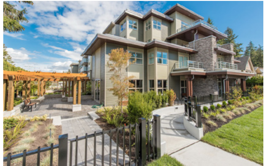
A seniors housing building with accessible design standards.
