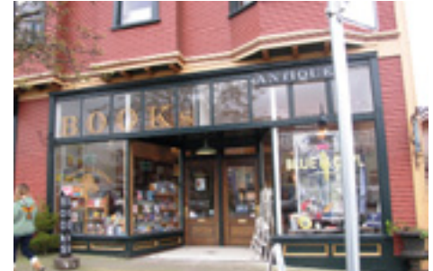
Recessed shop doors extend the window area for retail display and accentuate the shop entrance.
