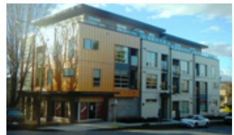
Changes in plane and variation of colours and materials reduce the overall building scale.
