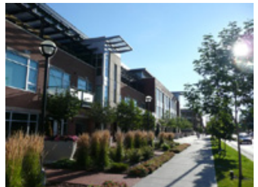
Beautifying the neighbourhood public realm can be achieved through good sustainable design practices that combine rainwater management and indigenous planting.
