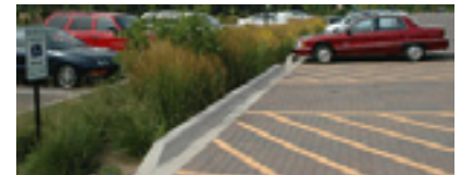
Permeable surfaces and landscaped areas or rain gardens are recommended rainwater management strategies.
