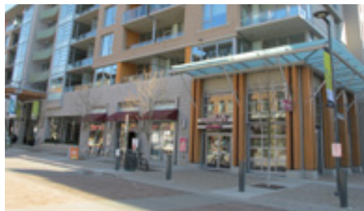
High quality materials, transparent shop fronts and unique signage and variety support walkability.
