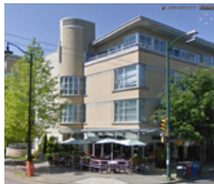
Roof overhangs and / or screening devices should provide weather and sun protection.
