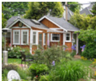
Gabled roofs, wood cladding, generous trim proportions, simple building forms and careful landscaping allow coach houses to fit into existing neighbourhoods and complement traditional and heritage style properties.
