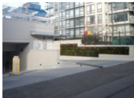
Landscape improves the appearance of underground parking access.
