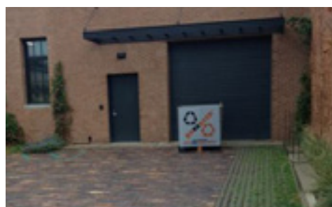
Rear elevations and parking lots should be attractive to neighbours who overlook them.
