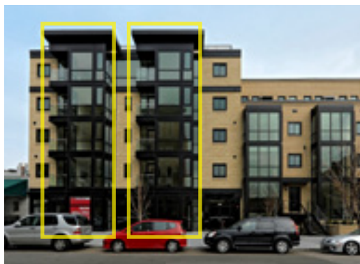
Varied roof forms and / or heights should relate to elements in the overall building form and massing.
