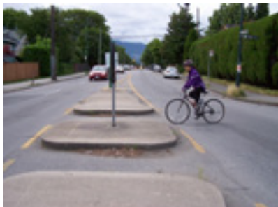
Example of two stage bicycle median crossing.
