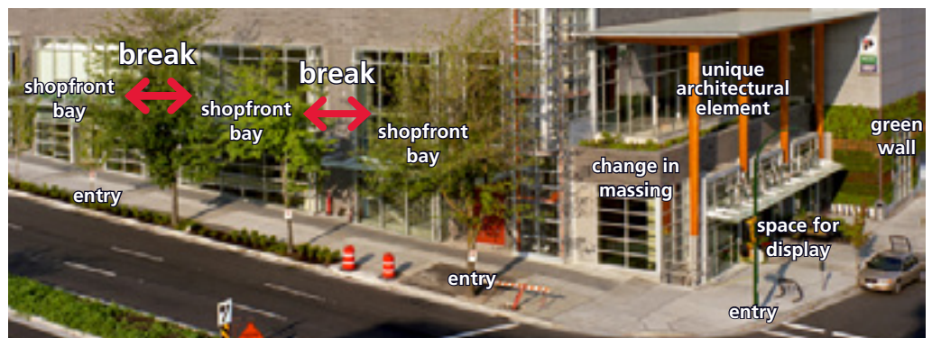
A number of strategies have been used to provide variation along this streetscape of two business frontages, including changes in material and plane, and variation in the design of weather protection, entrances and glazing patterns.
