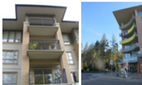
Materials, details and the form of balconies should be consistent with the overall building design.
