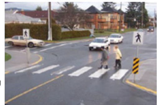
Example of a curb extension at an unsignalized intersection with signage and pavement markings.
