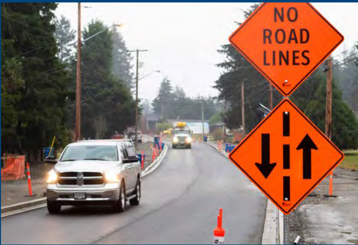
Metral Drive Complete Street Project
