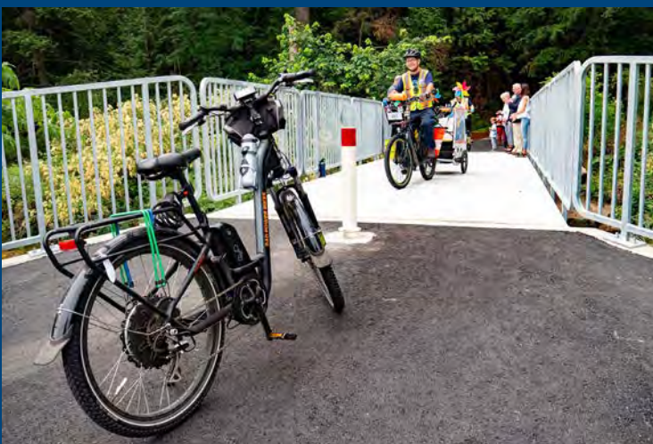
Lenhart Bridge Replacement
