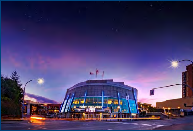
The Port Theatre - new roof
