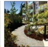
crushes gravel path
