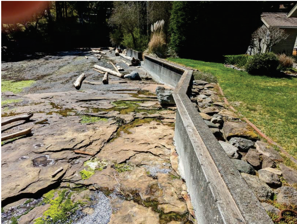
Photograph 4. View north – south along seawall forming natural boundary.
