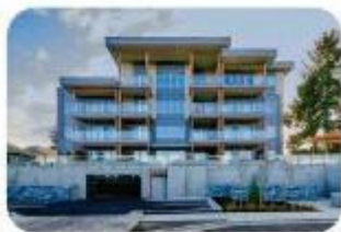
6010 Hammond Bay Road 53 Homes - Affordable Rental Housing
